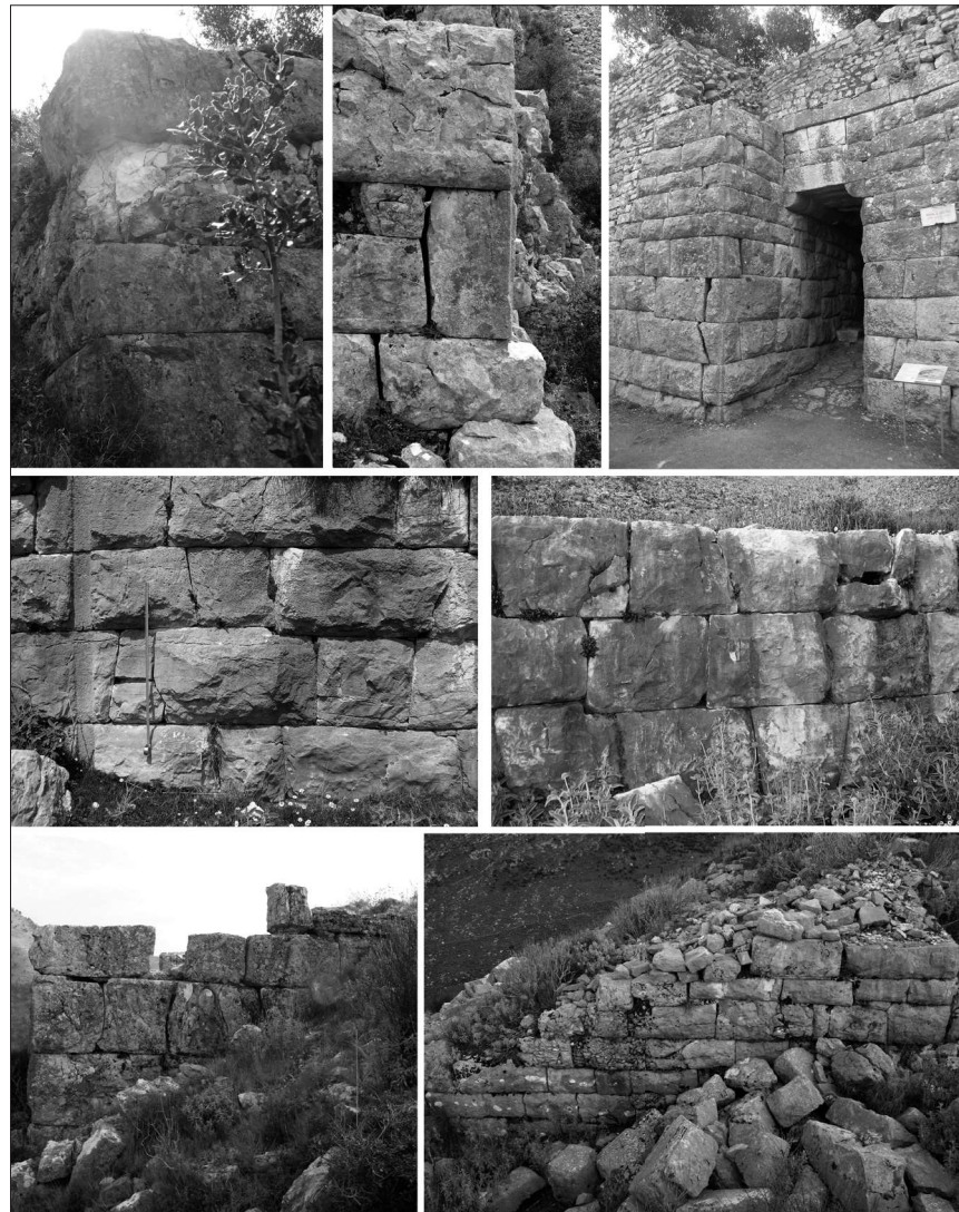
Fig. 14. Regular trapezoidal masonry: Selo (first two photographs), Butrint, Borshi, Hundësova and Malçani (last two photographs).
