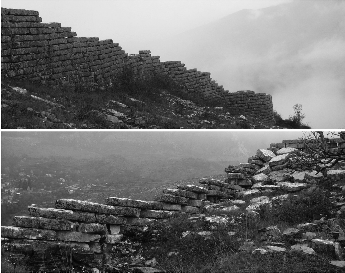
Fig. 12. Ashlar masonry at Paleokastra, near Labova: regular outer shell above and irregular inner face below.
